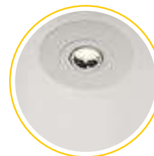
6. New recessed ceiling light placed into the reducer ring.
